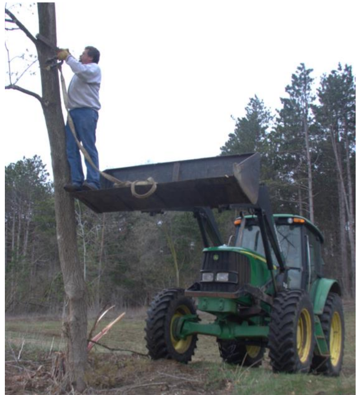
Dan Herum attached a strap as Eric Swenson prepared to persuade a box-elder from a line of trees removed west of Thrower #1. The removals should eliminate shadows for evening shooters.
