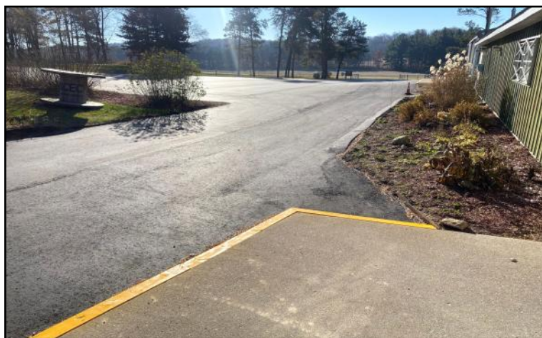
Members may notice a new north-to-south slope near the clubhouse front door, created to redirect run-off and save paving material.
